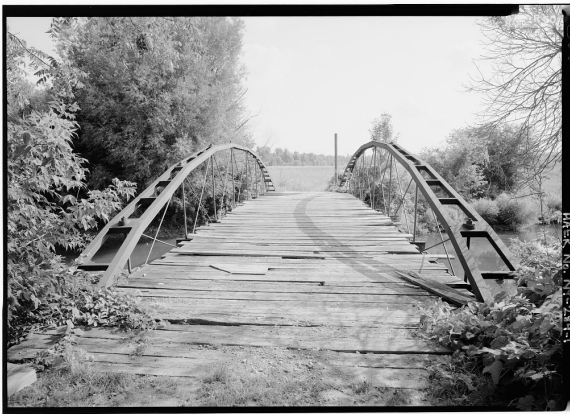
Figure 4. 1859 Ehrmentraut Farm Bridge. Photo by Jet Lowe 1994, Historic American Engineering Record (HAER).
