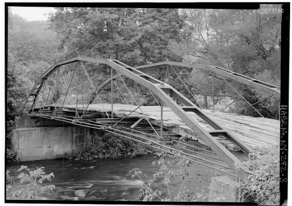
Figure 7. 1869 Vischer Ferry Bridge at Fonda before relocation to Vischer Ferry. Photo by Jet Lowe 1994, HAER.
