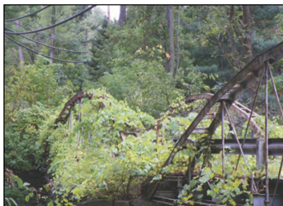
Figure 20. Shaw Bridge. Photo by Rick Ehrenberg 2010
