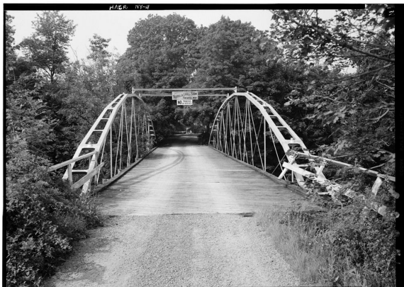
Figure 5. 1867 Normanskill Farm Bridge. Photo by Jack Boucher/David Plowden 1969, HAER.
