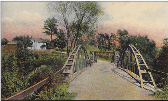
Figure 8. 1870 Shaw Bridge. Photo is from a circa 1900 postcard when the bridge was only about thirty years old.
