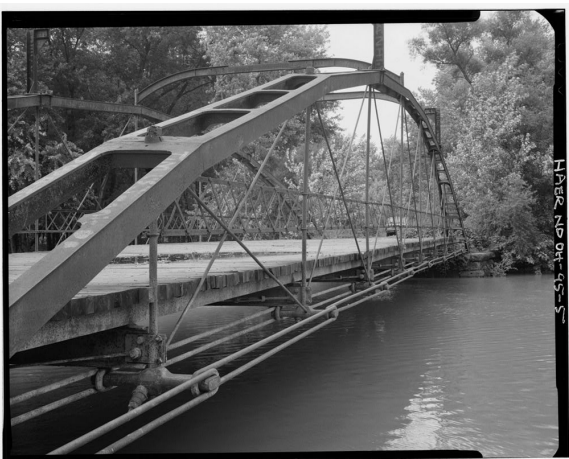
Figure 10. 1872 Rodrick Bridge over Wills Creek before relocation to Ohio State University Newark Campus. Photo by Joseph Elliot 1992, HAER.
