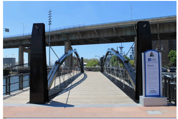
Figure 14. 2014 Commercial Street Bridge. Photo by Royce and Bobette Haley, 2016.
